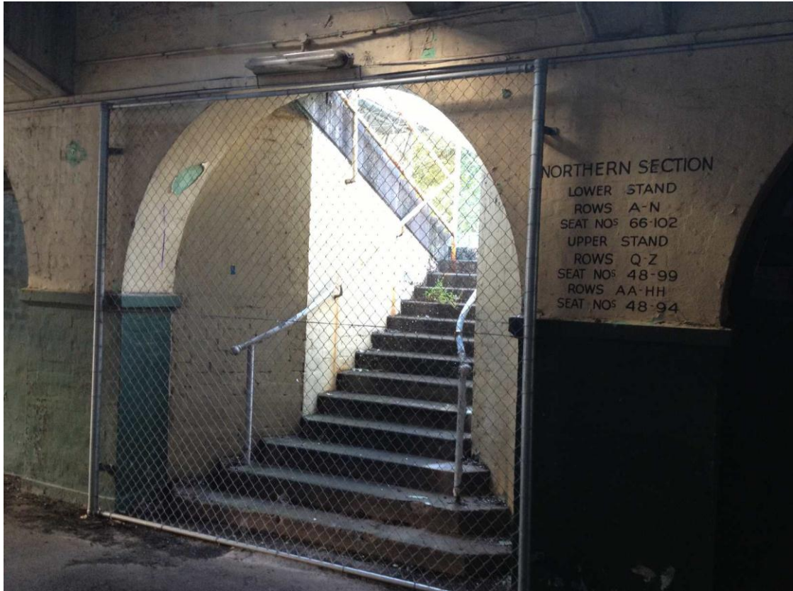
Figure 5. An arch beneath the northern grandstand providing access to the centre courts complex.
