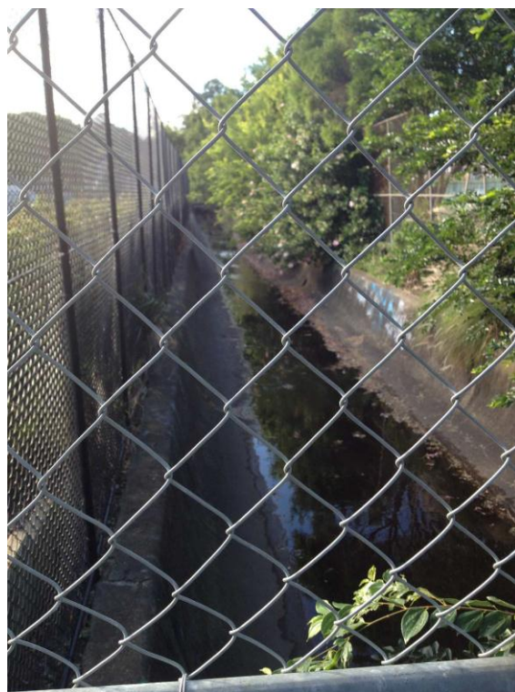
Figure 2. Storm water canal.
